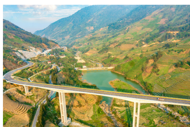
Coc San Hydropower Plant with a capacity of 29.7MW
