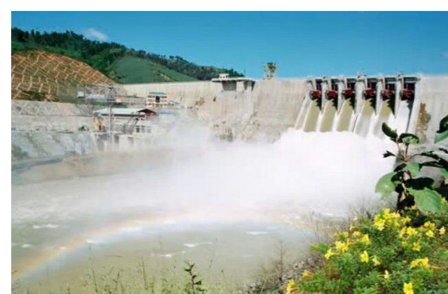
Ngoi Duong Hydropower Plant with a capacity of 11.4 MW
